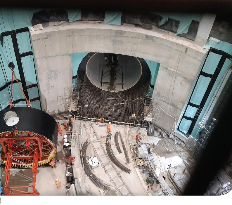
In addition to faster cycling, RCS MAX provided built-in leading-edge protection, an important safety provision as formwork units climbed seamlessly without needing to be repositioned at each level. Formwork engineers also incorporated a bespoke shoe adapter to maximise the width of influence, for high usage of the SCS system components and to support the specified concrete pressure, which resulted in an anchor load of 200kN.
